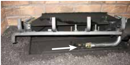
Diagram 2: Slide burner assembly to the right and then remove.
