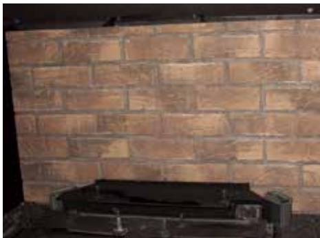
Back Panel Installed
