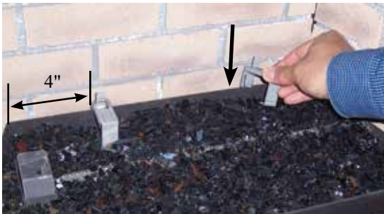
Brackets installed 4" from outside edge of burner tray
