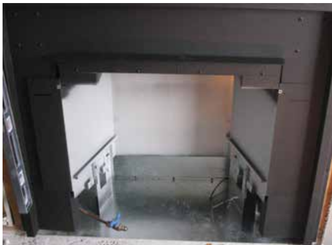
Outside firebox shown in position - refer to measurements (Step 7) before securing to surround.
