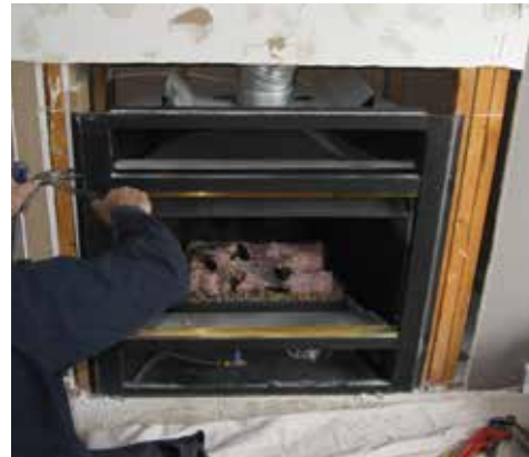
Remove unit from framing
