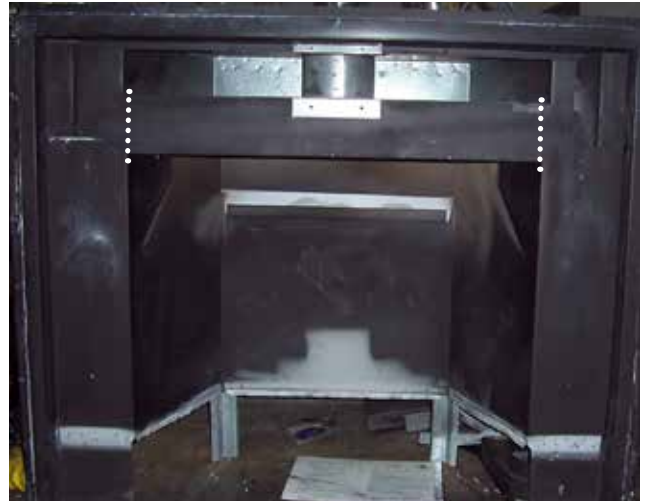
Cut out front cross piece to remove
