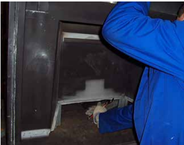
Flatten louver brackets
