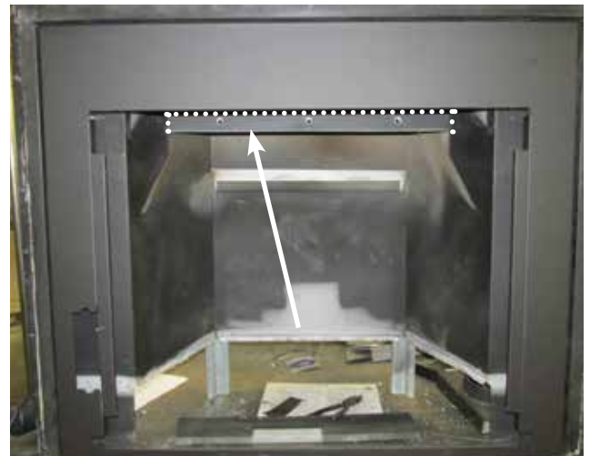
Cut out back cross bar
