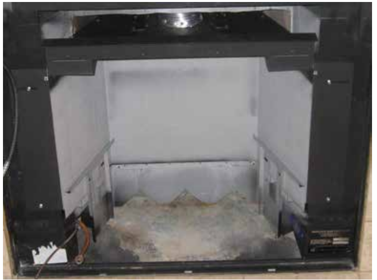
Diagram 7.14 Modified edges must be flush to allow proper seating of the E18E outerbox.
