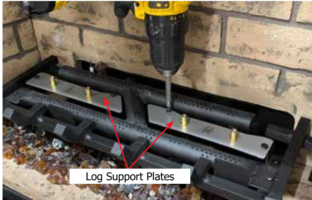
Diagram 5-Install Log support plate installation
