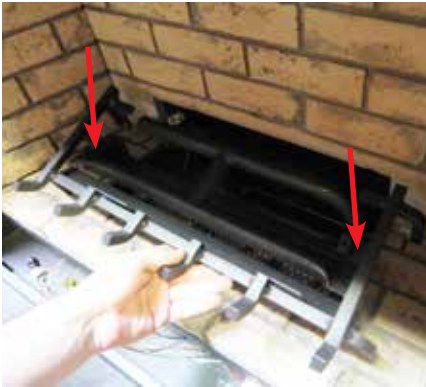
Diagram 1: Remove left and right screws.
