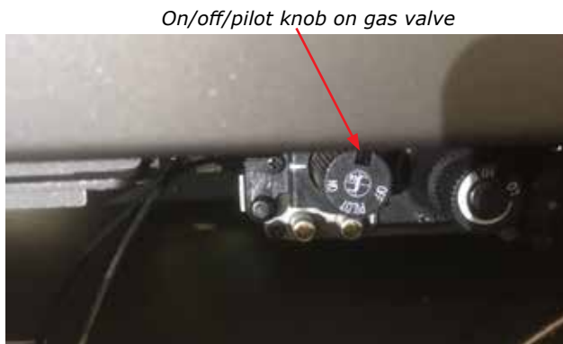
Knob extender slid over on/off/pilot knob on gas valve
