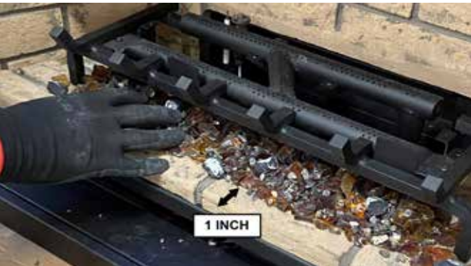
Diagram 4-Install Vermiculite + Lava Warning: Glass crystals must be placed at least 1" away from the front edge of the unit.
