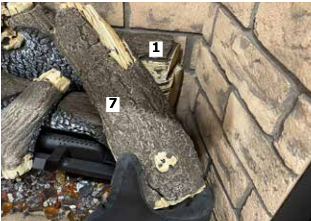
Diagram 12-Install Log 7
