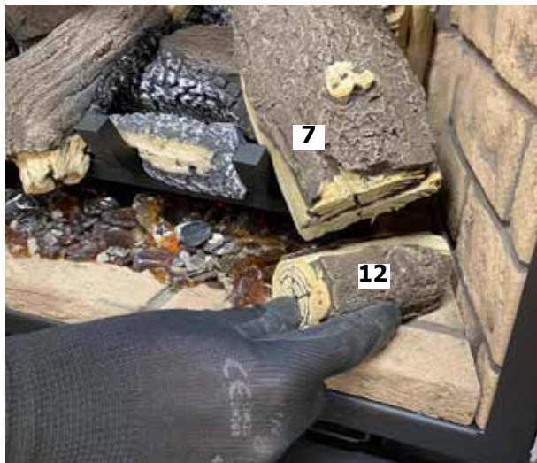
Diagram 17-Install Log 12
