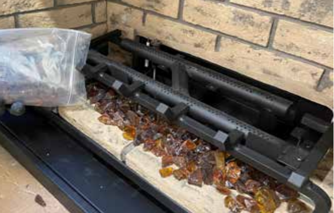
Diagram 3-Install Glass
