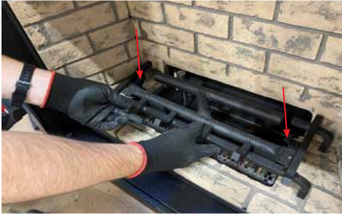
Diagram 2-Log Grate Install
