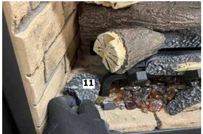
Diagram 16-Install Log 11
