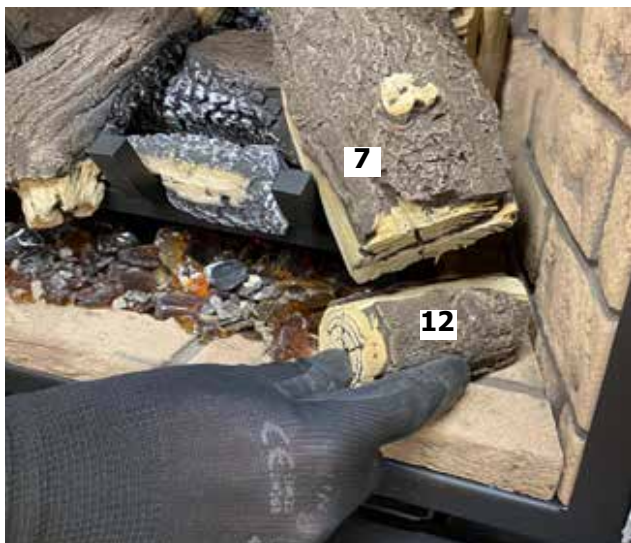
Diagram 17-Install Log 12
