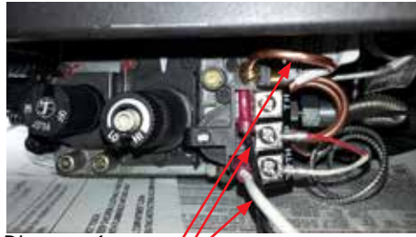
Diagram 4 Switch wires
