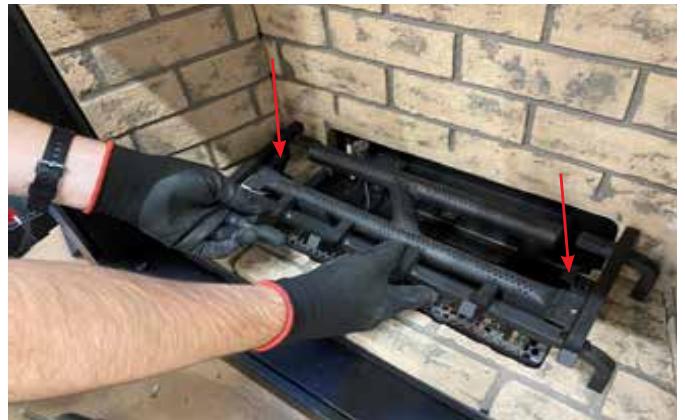
Diagram 2-Log Grate Install
