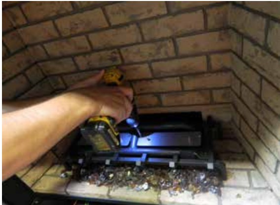
Diagram 5—Install Log support plates
