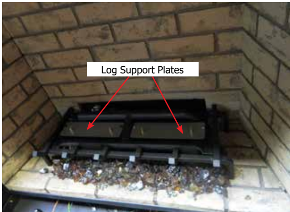
Diagram 6—Log support plates installed
