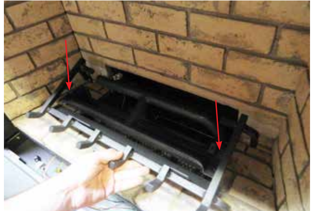
Diagram 2—Log Grate Install
