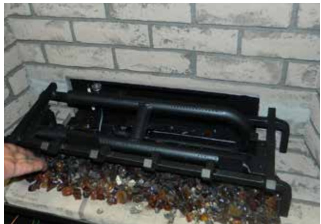
Diagram 4—Install Vermiculite + Lava
