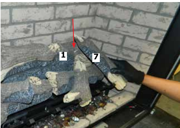
Diagram 13—Install Log 7
