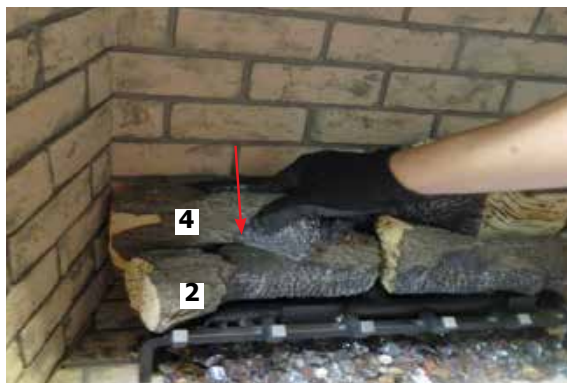
Diagram 10—Install Log 4
