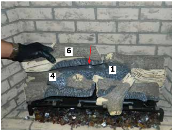
Diagram 12—Install Log 6
