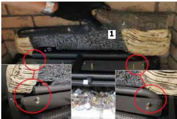
Diagram 7—Log 1 installation
