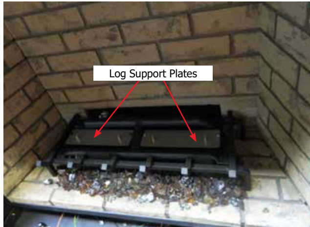
Diagram 6—Log support plates installed
