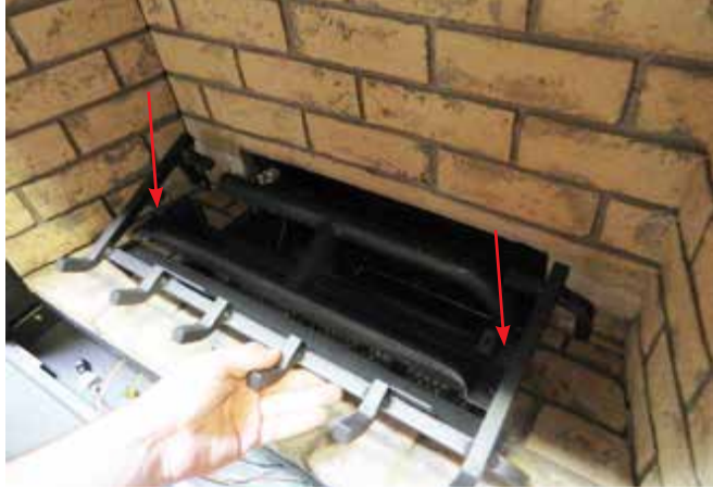
Diagram 2—Log Grate Install
