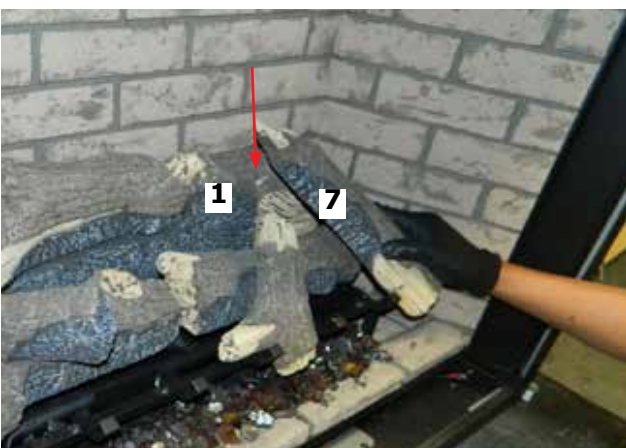
Diagram 13—Install Log 7
