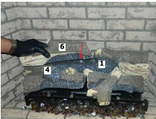
Diagram 12—Install Log 6
