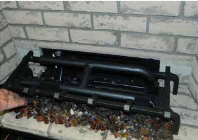
Diagram 4—Install Vermiculite + Lava
