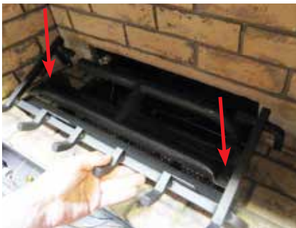
Diagram 1: Remove the left and right screws.
