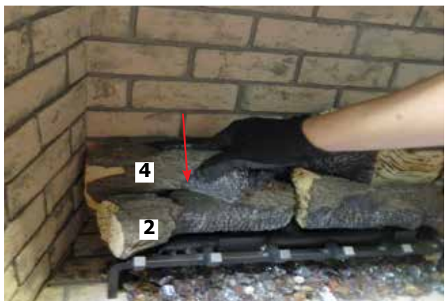
Diagram 10—Install Log 4
