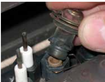
Diagram 2: Slide burner assembly to the right—then remove.
