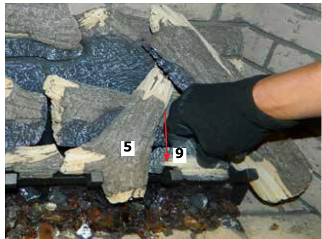
Diagram 15—Install Log 9
