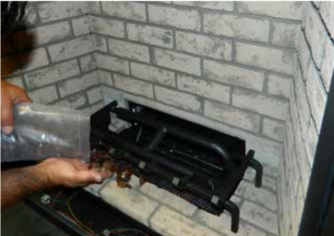
Diagram 3—Install Glass
