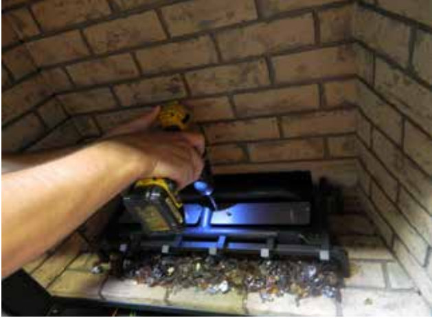
Diagram 5—Install Log support plates
