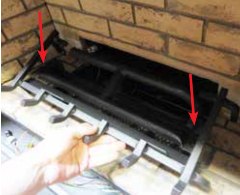
Diagram 1: Remove the left and right screws.
