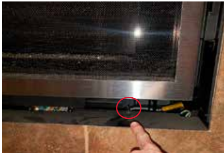
This Surefire switch is located at the bottom right center, behind the front wall.
