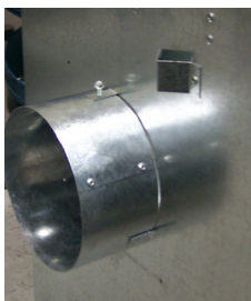
Center Round Duct collar over hole and attach to the tabs using 3 screws
