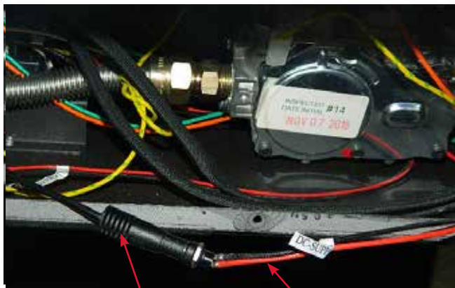
DC supply wire from wiring harness
